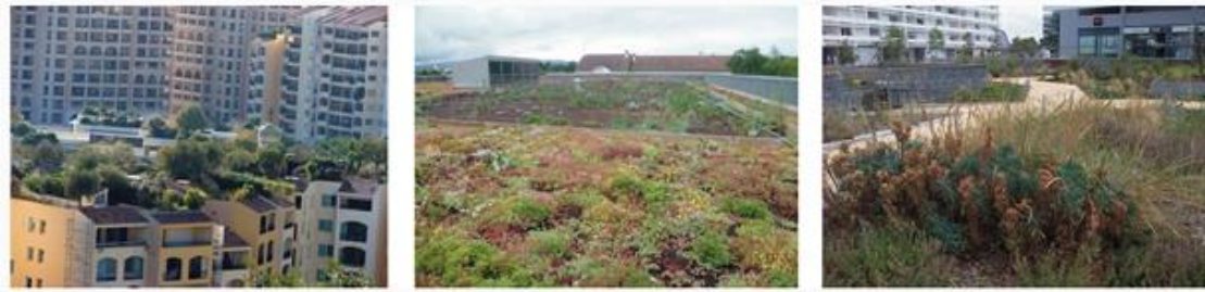
Intensive rooftop in Monaco (left), extensive rooftop in Dardilli France (middle) and semi-intensive rooftop in La Rochelle, France (right)
