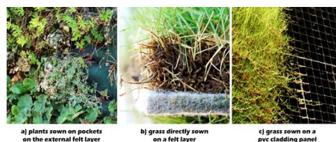
Different methods of plants attachment to the structure of extensive living walls (Mazzali et al., 2013)
