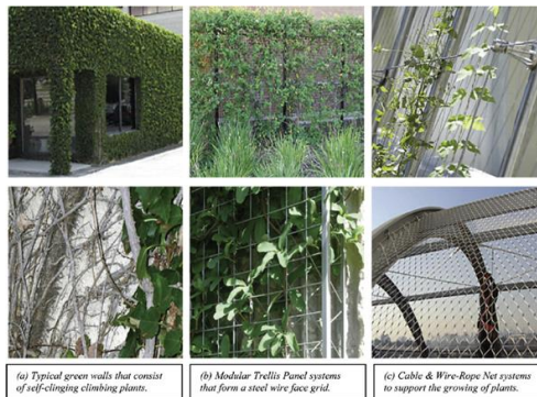
Facade greening system (Kontoleon and Eumorfopoulou, 2010)
