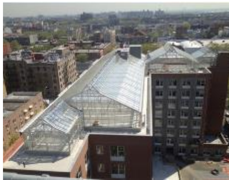
Greenhouse dak (nexuscorp.com)
