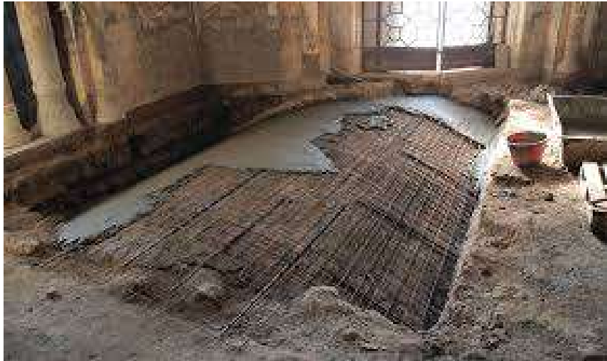
Reinforcement of a masonry vault.
