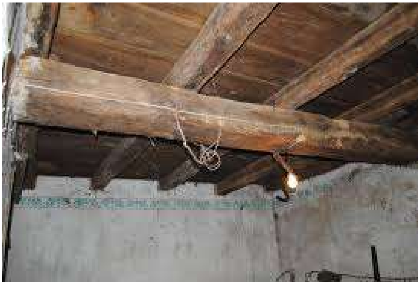
Wooden floor with main and secondary beams.
