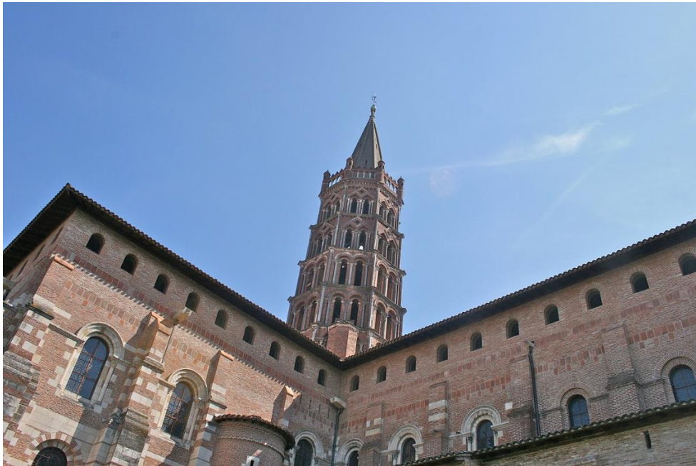
Figure: Under the roof of the nave and transept of the Saint-Sernin basilica in Toulouse, the mirandes restored during the "de-restoration" of Viollet-le-Duc's work © Mike Peel.
