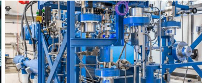
Gas Testing Laboratory
