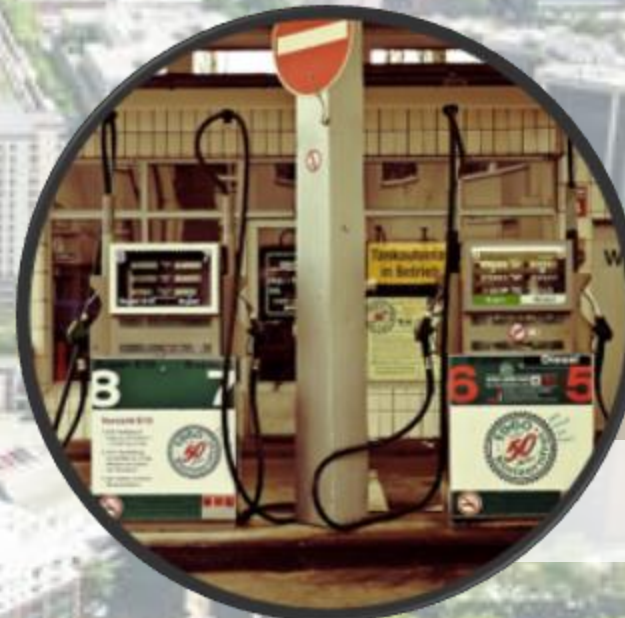
Leaky storage tank remediation
