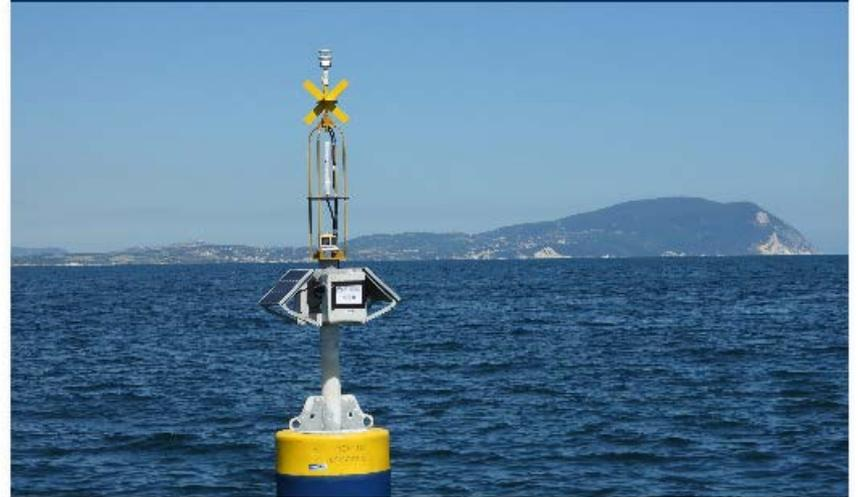
Marine weather station installed on a buoy near the artificial barrier of Porto Recanati
