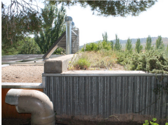
Figure 16. Plant rooftop in bioclimatic building cultivating aromatic plants, Centro de Agroecología y Medio Ambiente de Murcia, CEAMA, Bullas (Spain).
