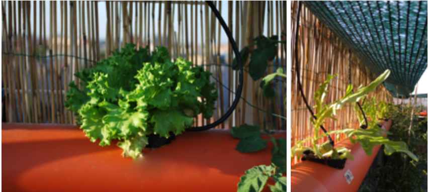
Figure 19. Shading structure in a public housing building rooftop garden, Bologna Italy.
