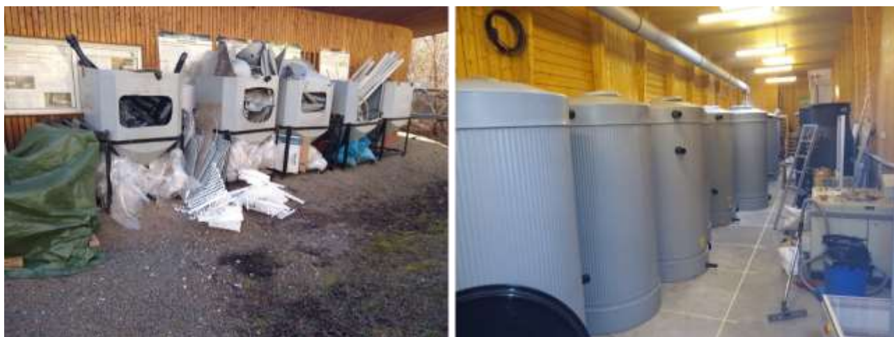
Figure 89. Conversion from the old to the new wastewater recycling plant. The old tanks have been removed and are now being recycled (left). The new tanks arrived and were placed in the water house to complete their installation.
