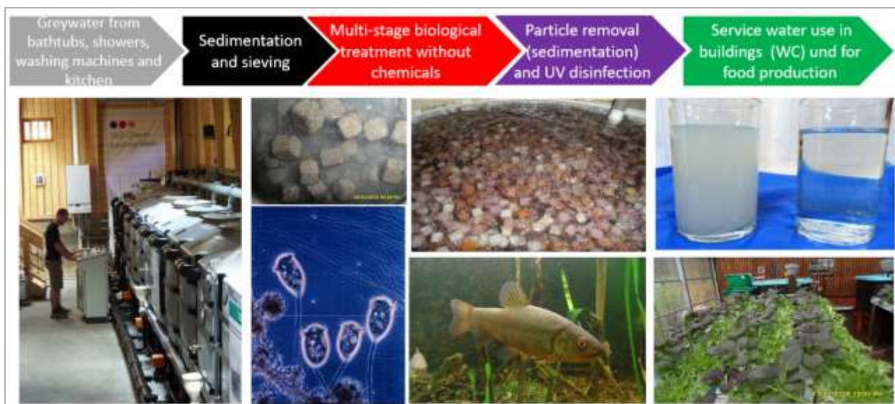
Figure 87. The existing water recycling plant in the "Water House". The water is purified purely biologically using microorganisms without the addition of chemicals, so that the water can ultimately be used for vegetable production and fish farming.
