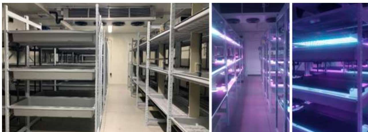
Figure 12. Structures for layered production (left), equipped with LED lighting system (Flytech Srl) (right) of AlmaVFarm.
