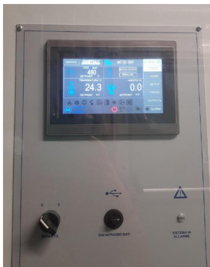
Figure 20. The interface of the heating, ventilation, and air conditioning unit (HVAC) of ALMA VFarm.
