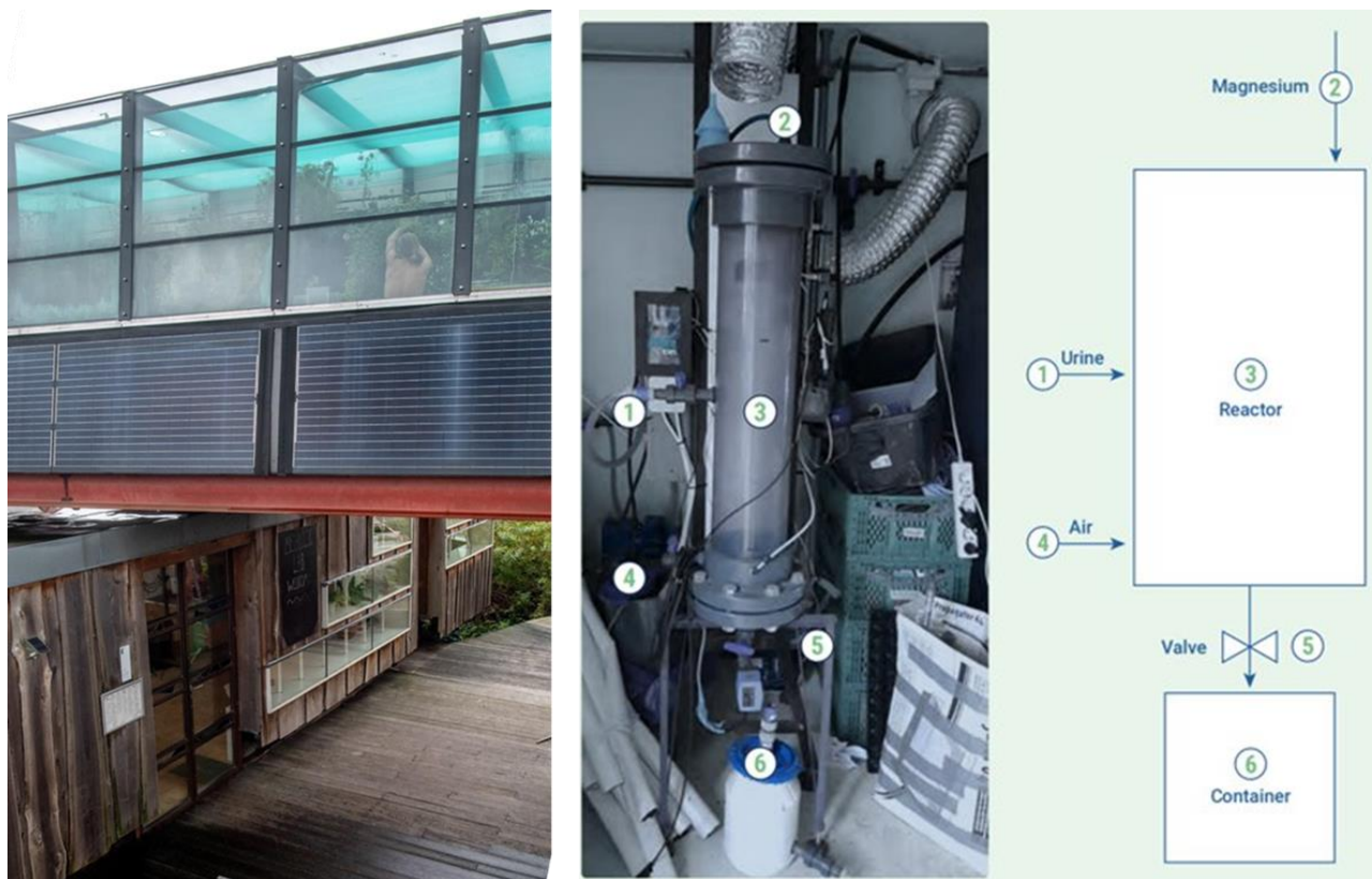
Figure 64. Metabolic aquaponic farm (left) and semi-automated struvite reactor connected to the sewers system, below the farm (right).
