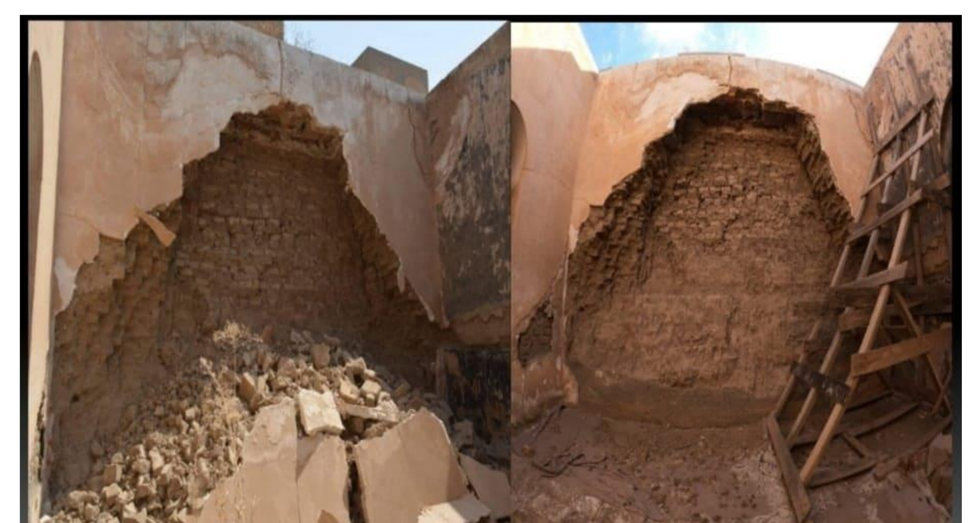
Collapses in the courtyards of Nabu-shkhari Temple
