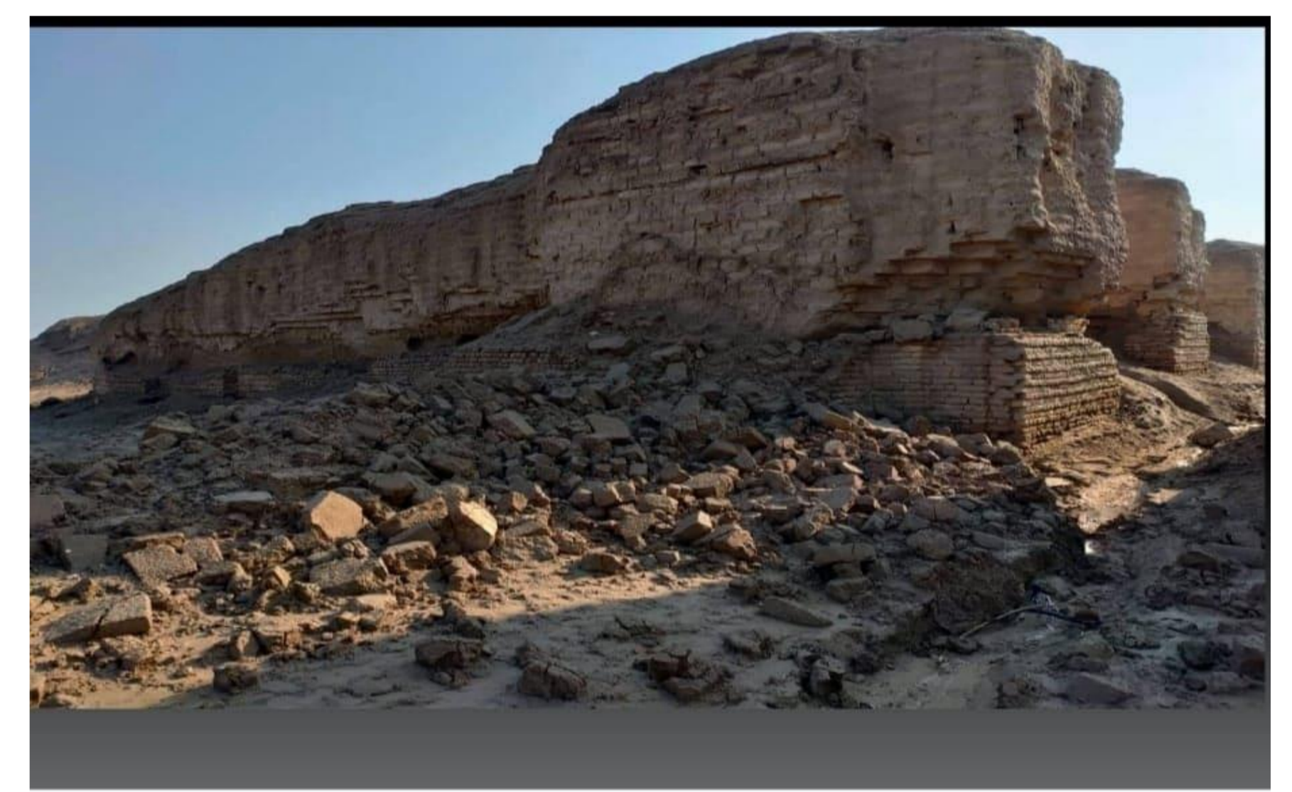
The facade of Ishtar Temple at Kish
